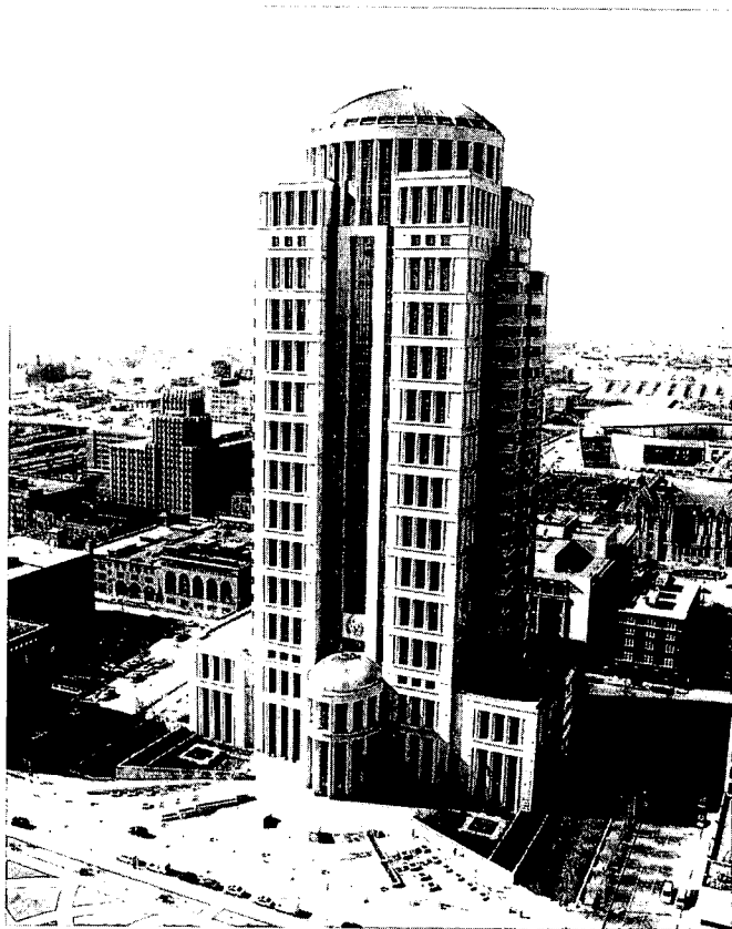
FIGURE 24. Thomas F. Eagleton Federal Courthouse . St. Louis, Missouri. Architects: Hellmuth, Obata + Kassabaum, Inc., 2000. Photographer: The Honorable David D. Noce, Magistrate Judge of the Eastern District of Missouri. Photograph courtesy of and reproduced with permission of the photographer.
